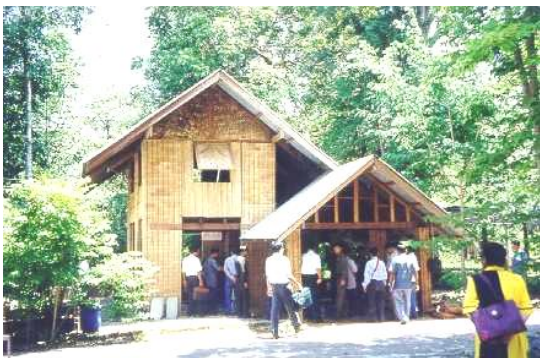
First blockprasan's housing build in B.E. 2527
